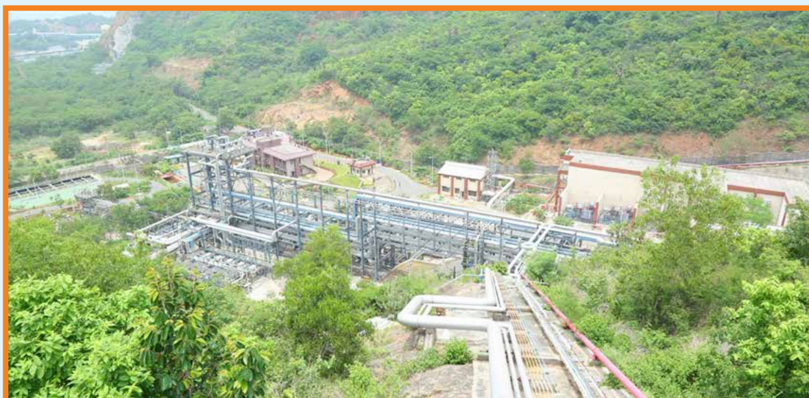
Aerial view of Vishakhapatnam Site
