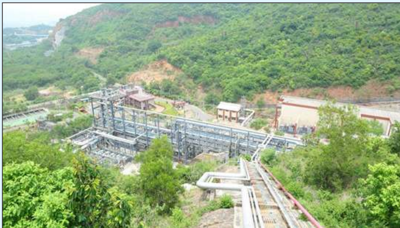
View of the aboveground facilities at Visakhapatnam
