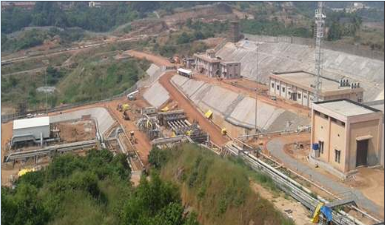
View of the aboveground facilities at Mangalore
